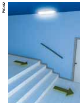
Near the stairs so that each step receives direct light.
